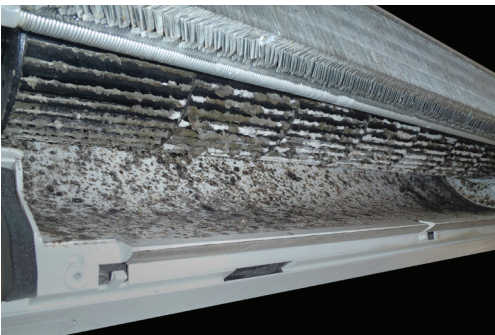
Mold thrives on mini-split blower wheels
